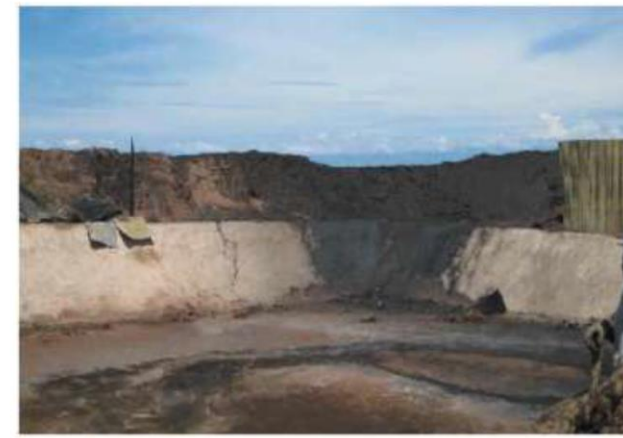
Photo 6: the damaged flare pit following the Kingfisher-1 well test, showing damaged steel sheets
